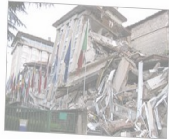
Earthquake damage to the Hotel Degli Abruzzi in L'Aquila.
