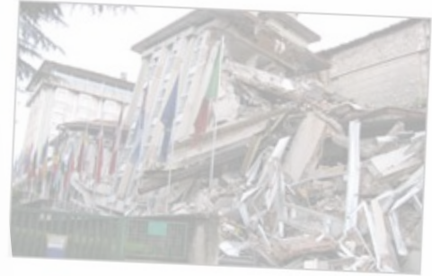
Earthquake damage to the Hotel Degli Abruzzi in L'Aquila.
